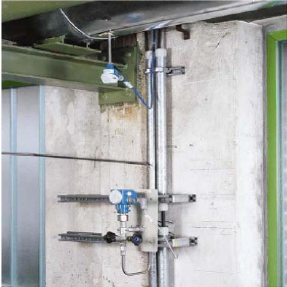
The graphic above shows a field installation for controlling temperature and pressure of steam in the low-pressure system. These are process inputs for controlling the regulating valve. The head mount temperature transmitter is used in conjunction with an integrated temperature sensor assembly.
